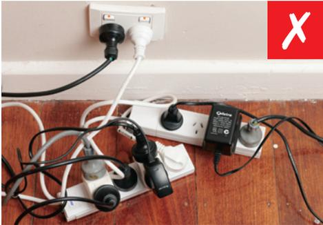
A double adaptor or a powerboard plugged into another double adaptor or powerboard creates a danger of overloading the system. For safety, use a single extension cord rather than joining shorter cords. Leaving an extension cord coiled while in use or placing a cord under floor coverings can cause overheating.
